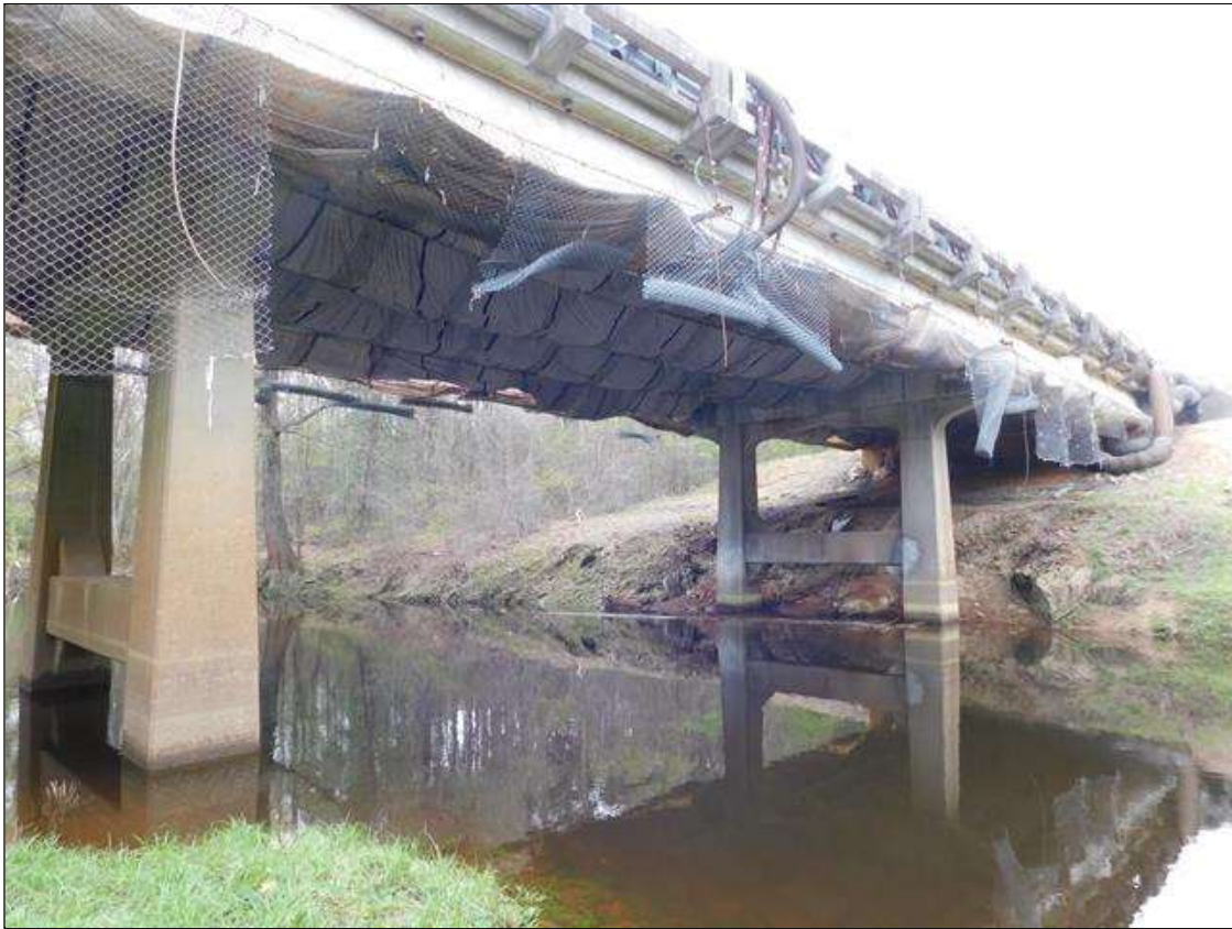
Upstream profile, looking East
