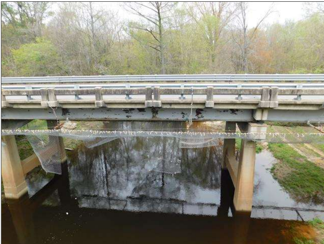
Upstream view, looking West
