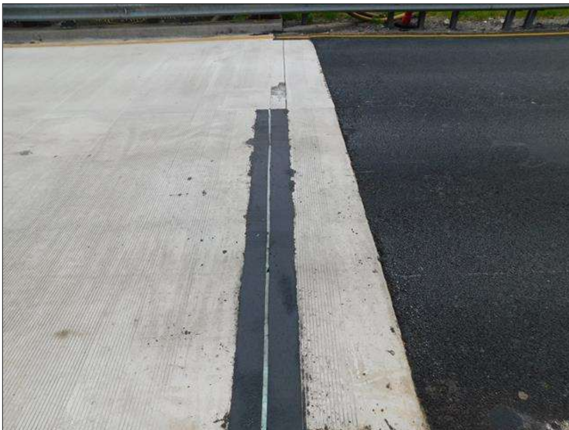
End Bent 2 joint
