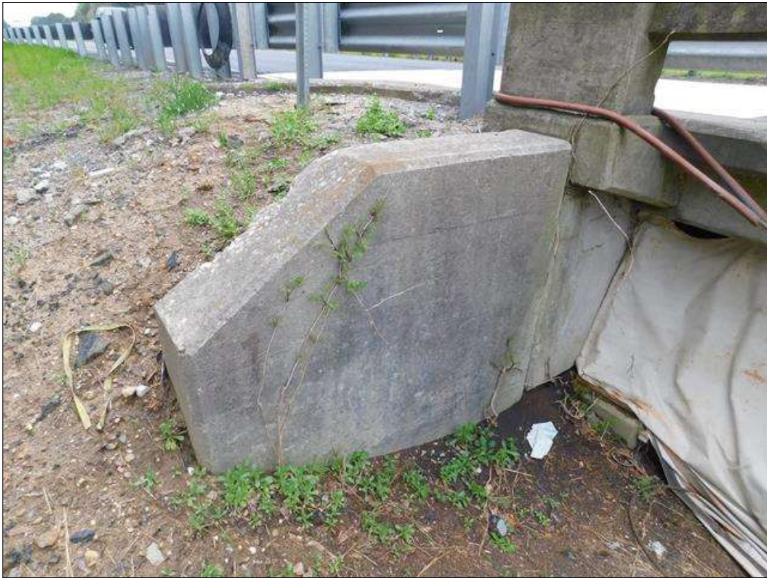
Southeast wingwall (All others similar)
