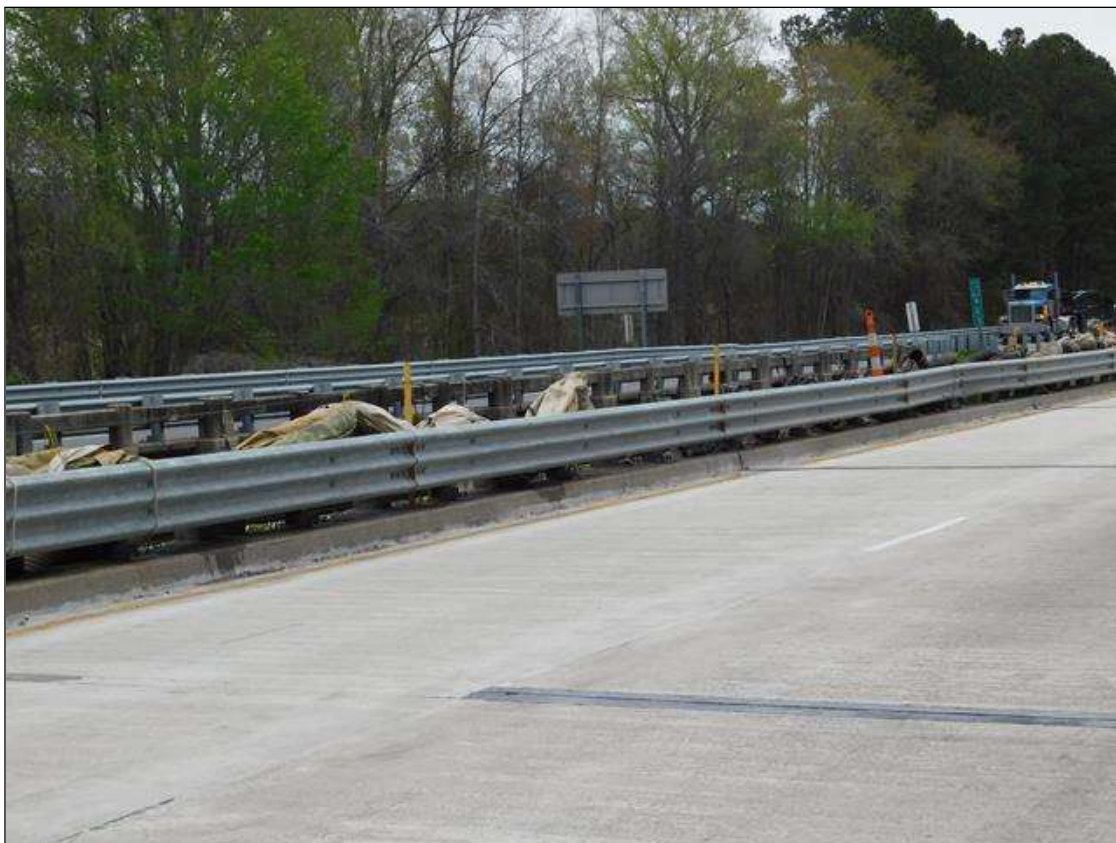
West bridge rail (East bridge rail similar)
