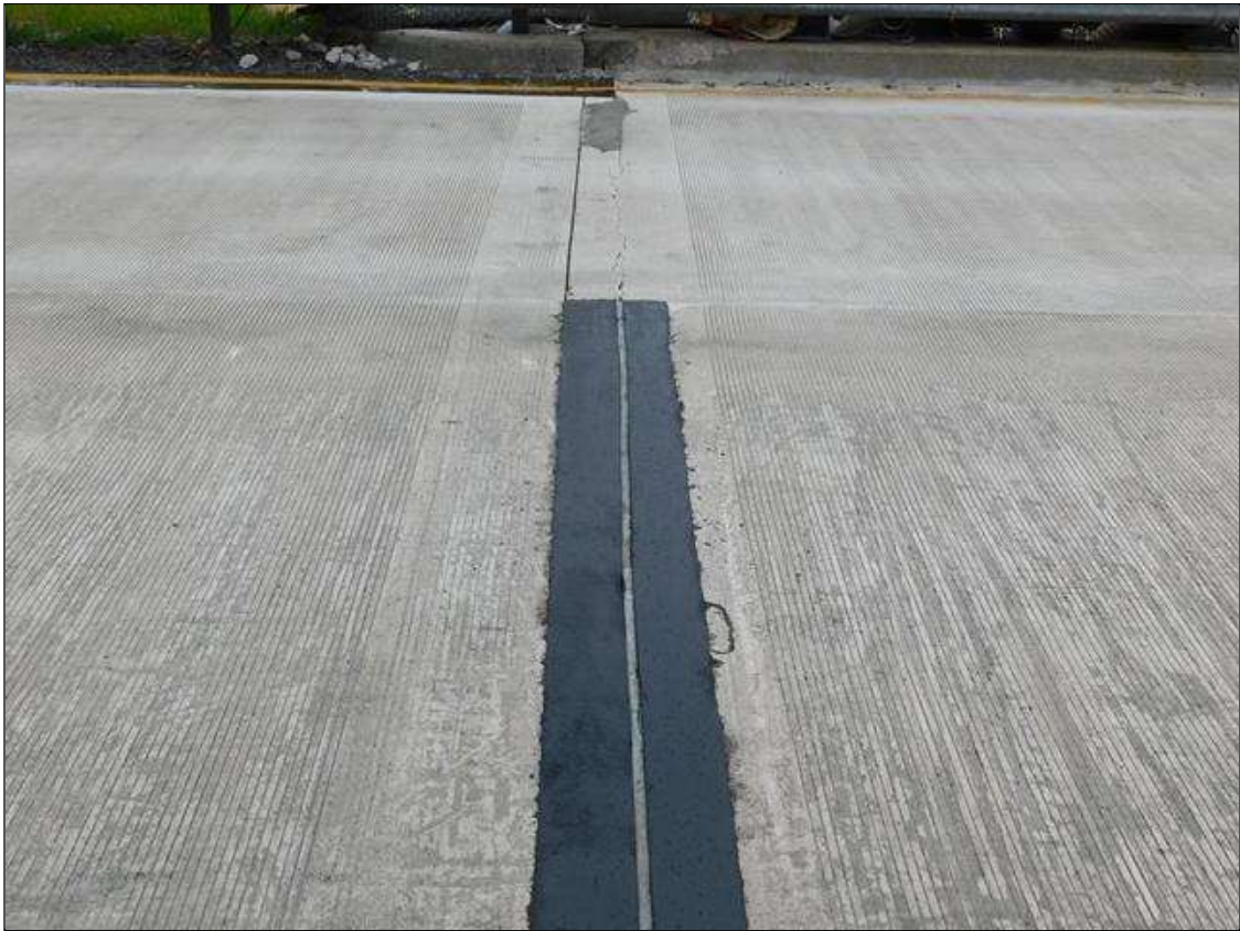
End Bent 1 joint
