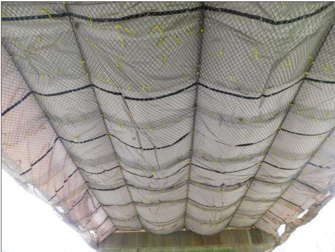
Underside of superstructure (Span 3 shown)
