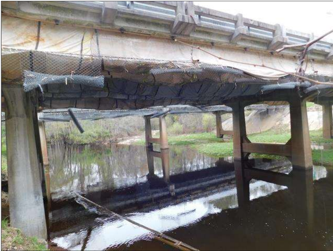
Downstream profile, looking West
